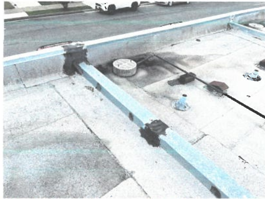
Figure 8. Past leak repairs..
