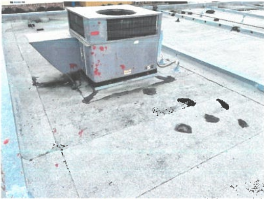
Figure 7. Past leak repairs...
