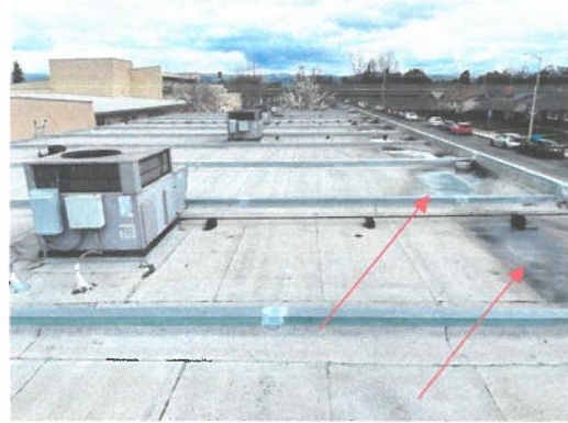
Figure 2. Ponding water along the low eave.
