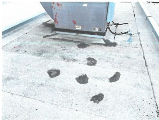
Figure 6. Patching of the roof.
