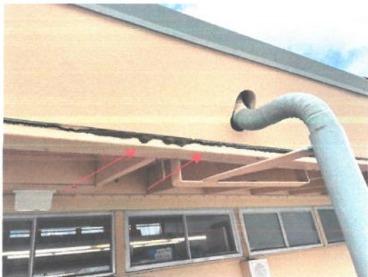
Figure 12. Moss growing from water intrusion...
