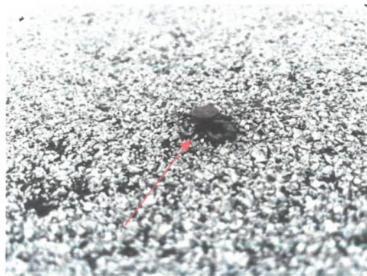
Figure 4. Nails from the plywood decking backing out through the roof.
