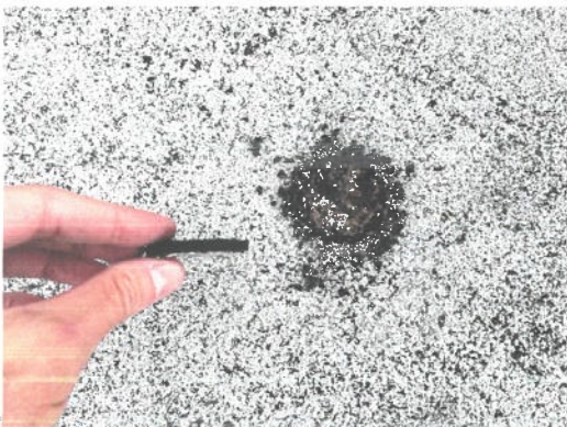
Figure 3. Thin & fragile roof membrane.
