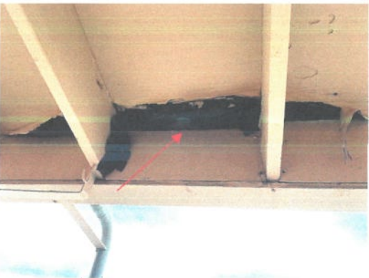
Figure 11. Damaged plywood decking from long-term leaks.
