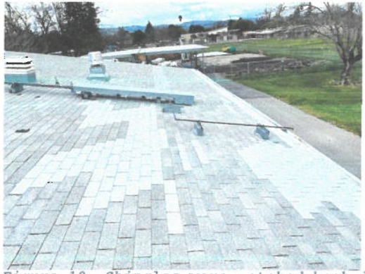
Figure 10. Shingles were patched back in 2005/06
