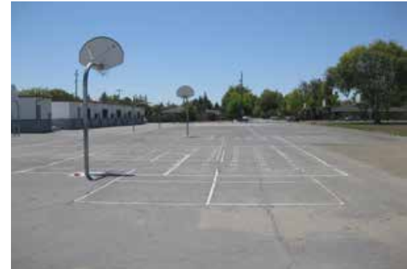
Typical AC paving at hardcourts
