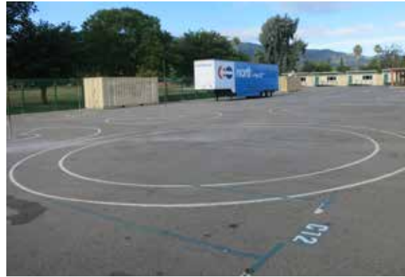
Typical AC paving at hardcourts
