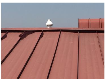
4. The gaps have become very large along the ridge, allowing for wind driven rain to infiltrate under the metal panels. Also noted was the ridge cap was not riveted to the zee closures (improper installation).
