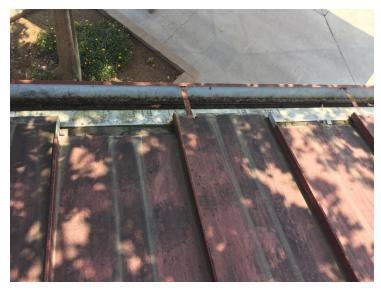
3. The panels are buckling at the ridge resulting in damage to the zee closure and ridge cap.
