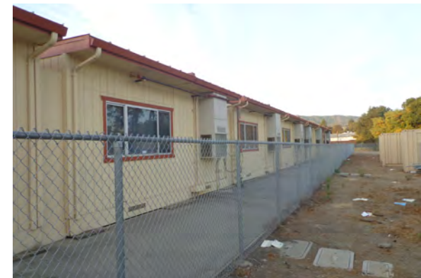
Typical portable Bard units
