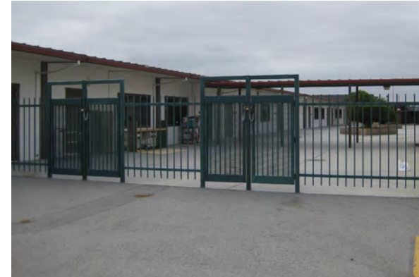
Typical steel ornamental fencing and gates
