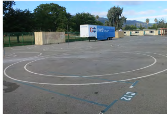
Typical AC paving at hardcourts
