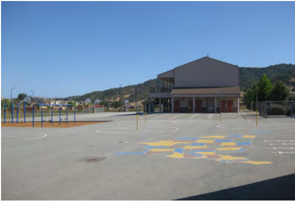
AC paving at hardcourts
