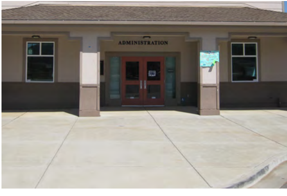
Typical concrete paving
