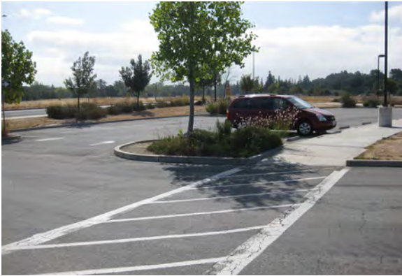
AC paving at parking area
